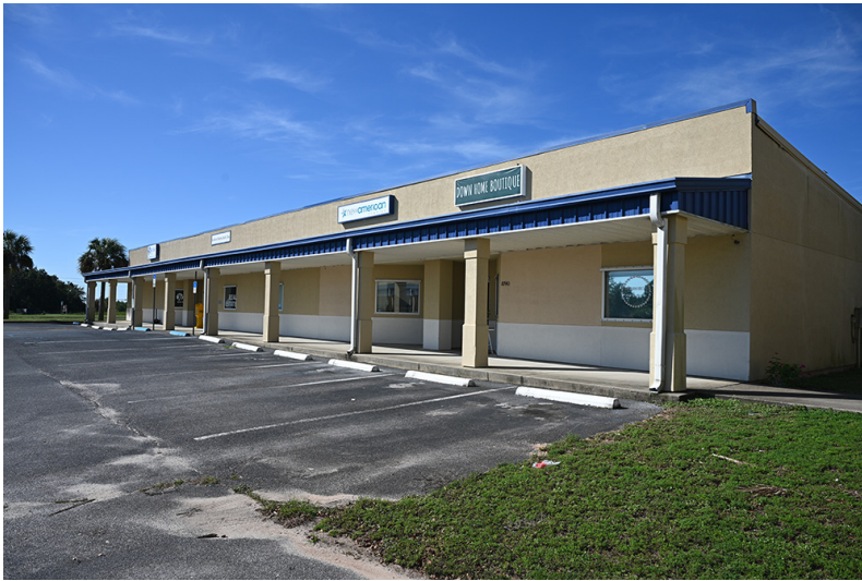
Looking at Building 2 – southwest view
