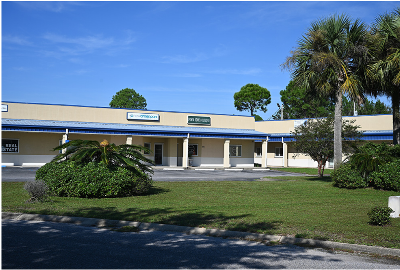
Looking northwest at Buildings 2 and 3
