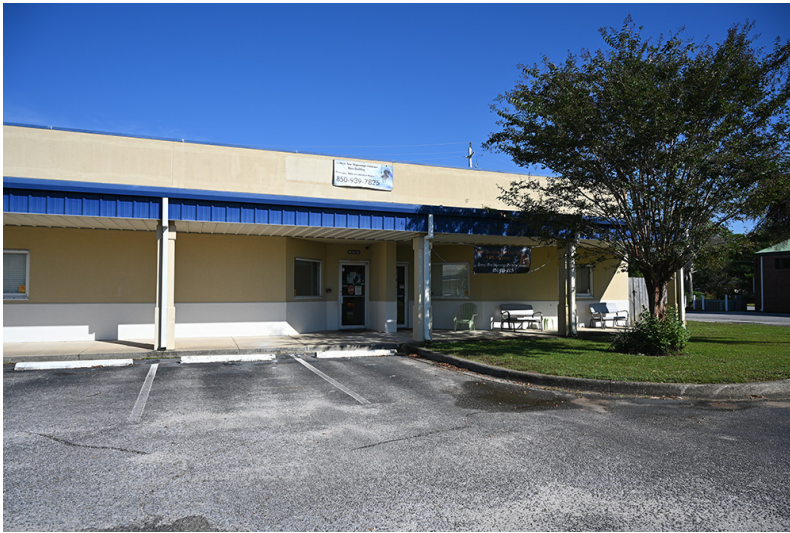
Eastern side of Building 1
