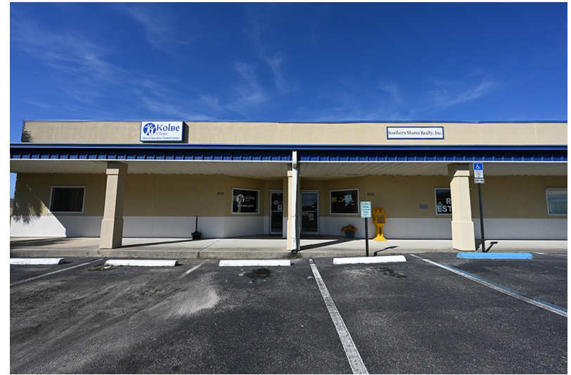
Most southern side of Building 2
