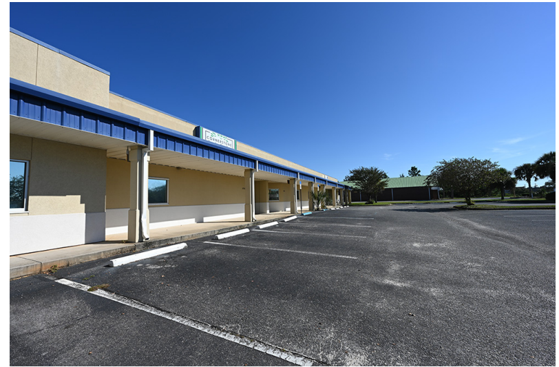
Building 1 looking east to west
