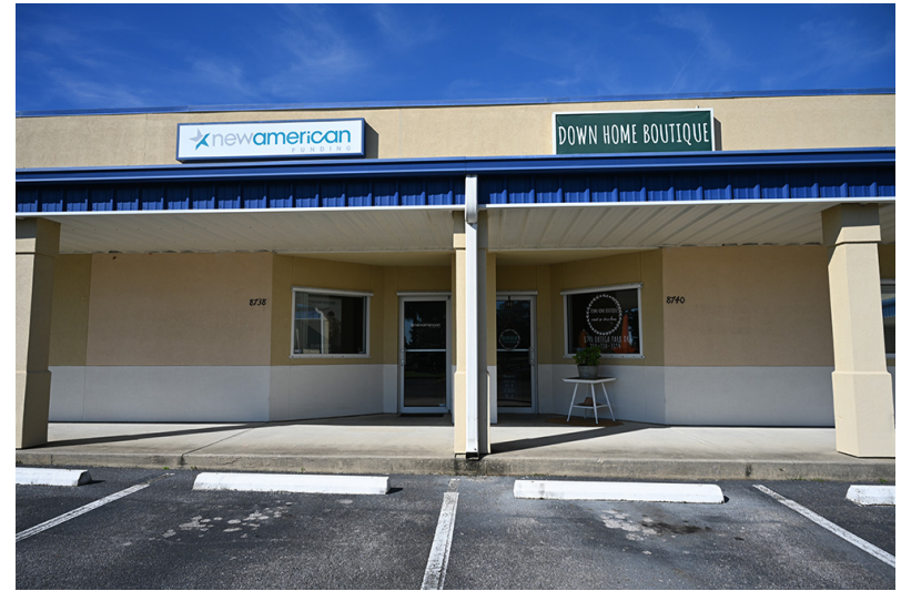
Northern side of Building 2
