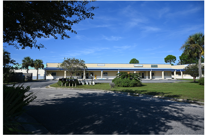
Looking east at Building 2.
